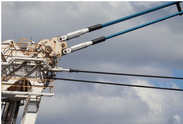
Figure 2. Applied Fiber main and IBS pendants at Tri Structure.
